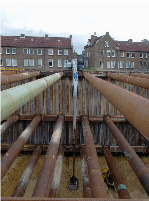
Figure 2. Application of OM in Maastricht for A2Maastricht tunnel (photo Reen van Beek)
