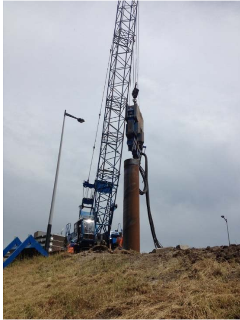
Fig. 6: Vibro driving of steel piles on top of the embankment
